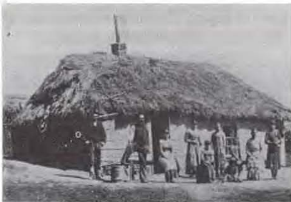
A Sod house of the early eighties, with thatched roof. Madison county, Nebr. (From an old print).
