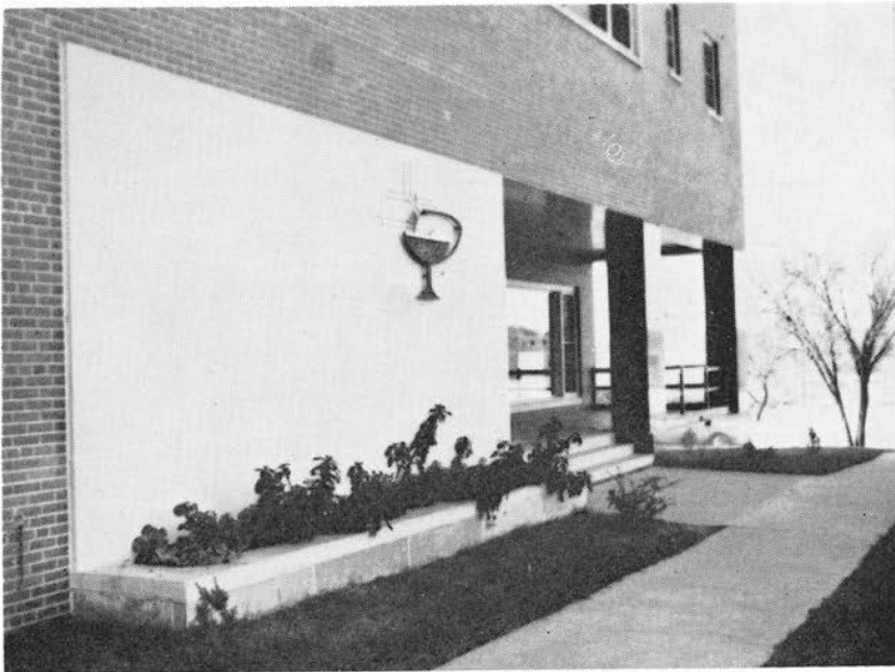
School of Nursing Building
